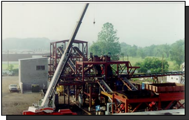
Installation of modular briquetting system
