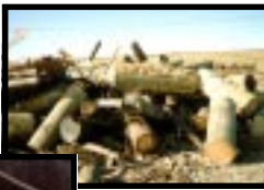
C & D Debris
