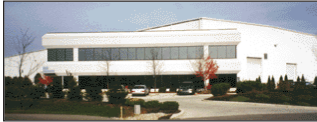
45,000 sq. ft. engineering & manufacturing facility in Groveport, Ohio.
